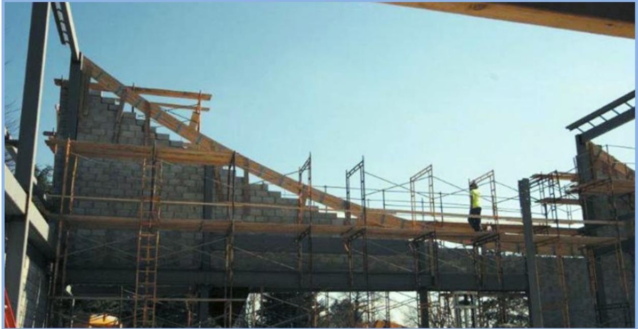
Figure 2: Concrete Bond Beam Form
